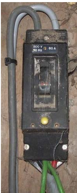
60 A voltage-operated earth-leakage circuit-breaker
