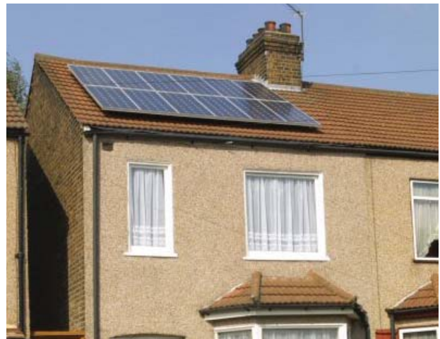
Photovoltaic installation (photo courtesy Energy Saving Trust)
